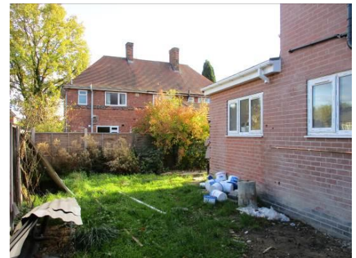
Rear garden towards nos.33 and 35 Brook Road
